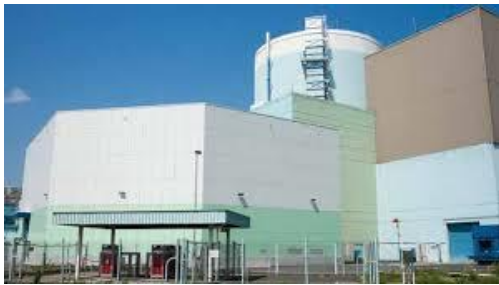
Nuclear Power Plant (NPP) Krško
